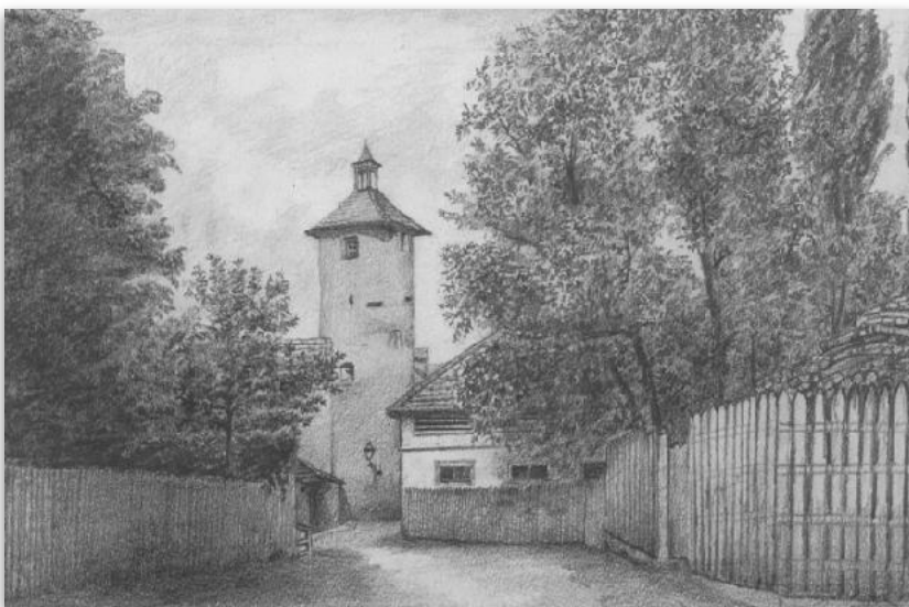
The drawing by Henri Baudinot (1869-1926) shows the Bollwerk tower. On the left the palisade surrounding the cemetery ; on the right , the slaughterhouses
